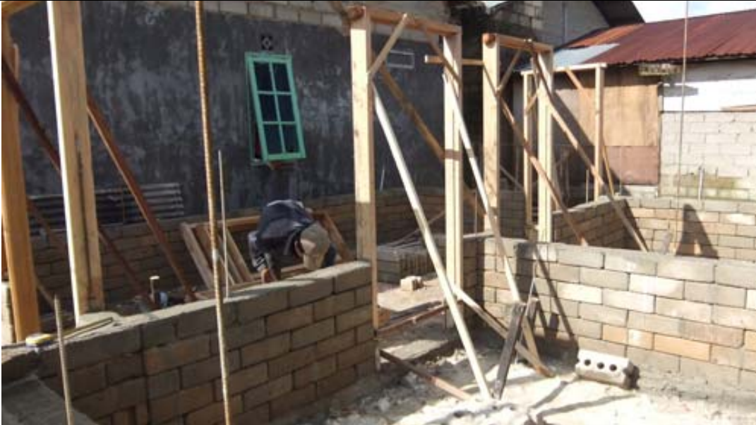
Above: The Interlocking Brick house under construction
